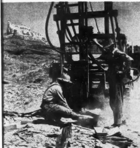
ABOVE: The deep hole percussion drill is a new exploration tool. BELOW: Every mine car of ore counts in the atomic energy age.
